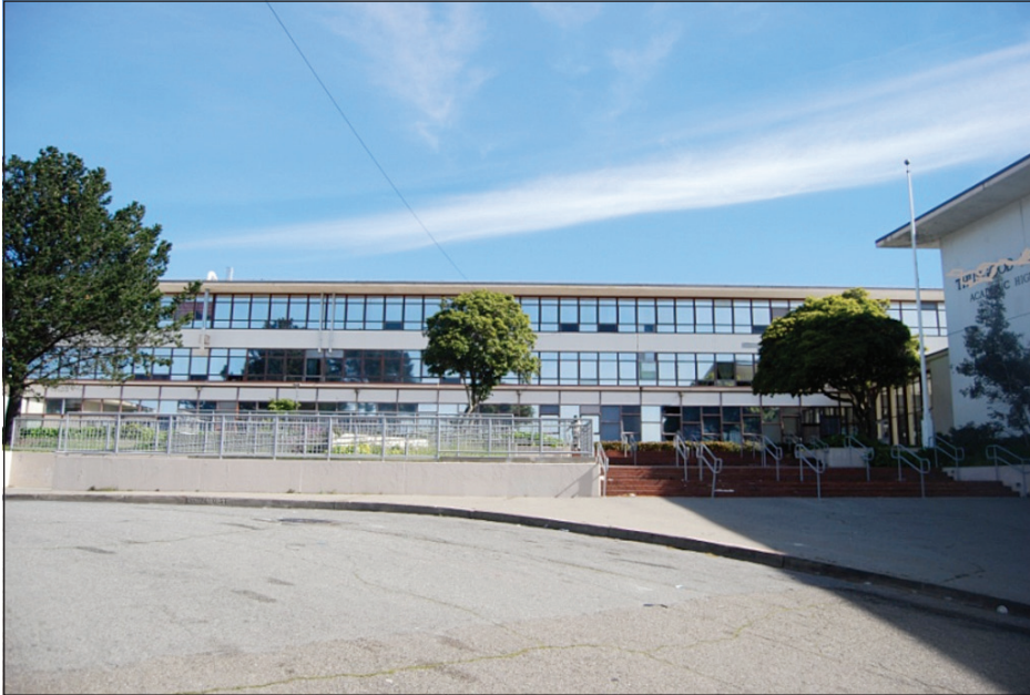
Figure 2-11: Urban high school in inner-city residential neighborhood of single-family houses
